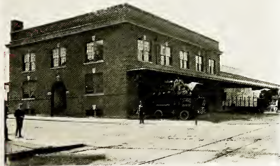
Pennsylvania R. R. Freight Station Pennsylvania Ave. and Northampton St.
